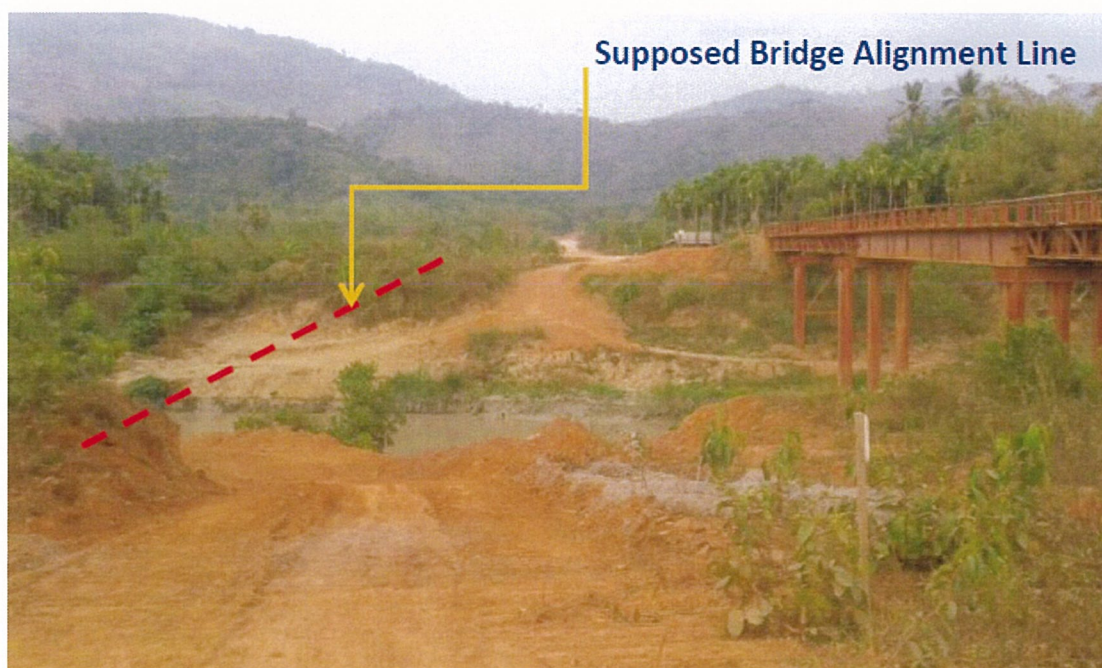
PHOTO 4.2-2 : TALAING YA CHAUNG AT STA. 19+271
