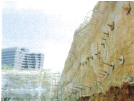
Soil Nailing Application
