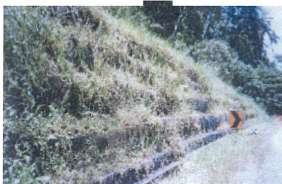
Gabion Wall Together with Grassing
