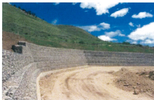
Gabion Retaining Wall of Back Slope
