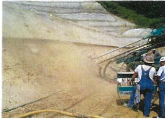
Soil Nailing Construction Techniques
